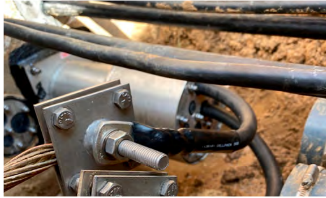
Special construction of a building earthing for transmission system operators
