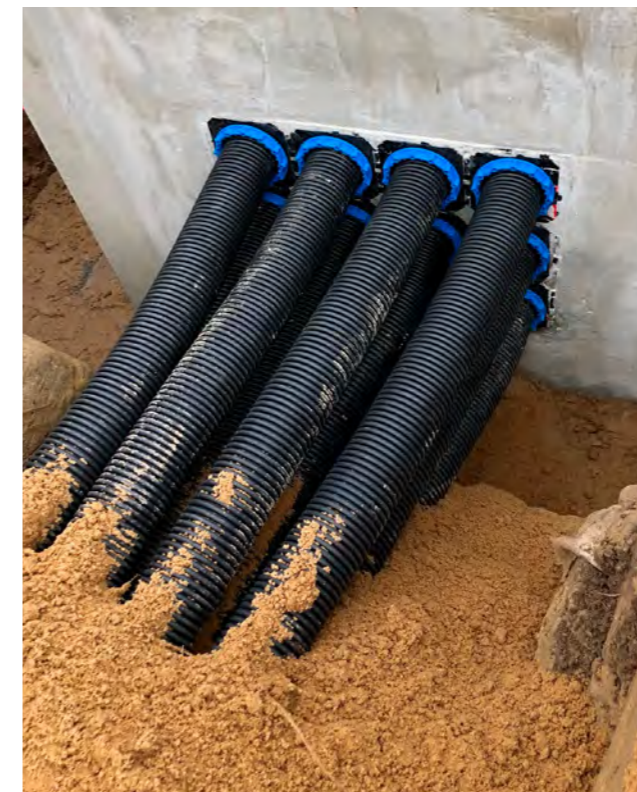
KD110-K2/3x4/(L) with system cover KD110-D-DGM110
