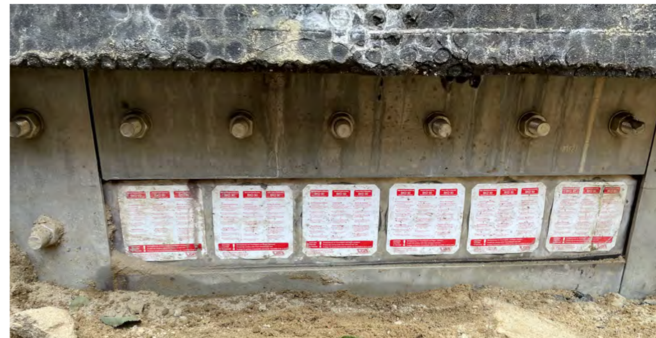
BKD 90 with fixed and loose flange design
