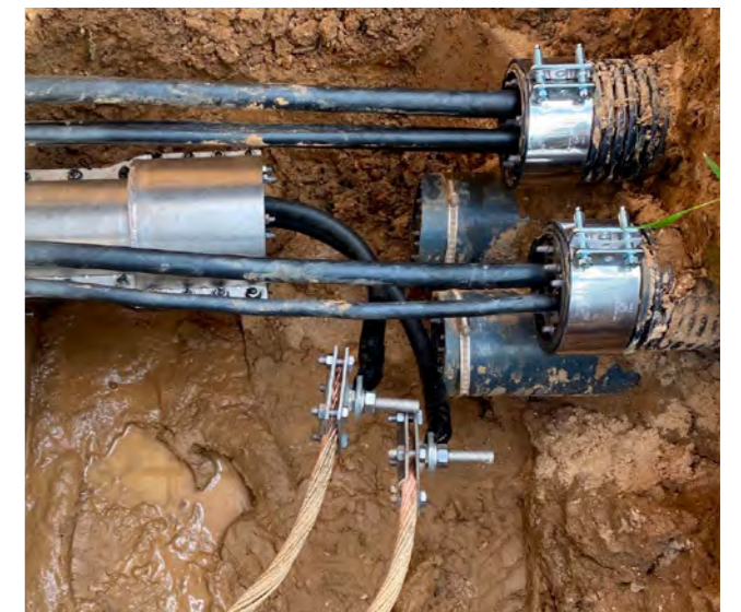
GPD-CV93/G/60/WE50/V2A/EPDM/ (Z)x(D): for sealing exposed corrugated pipes
